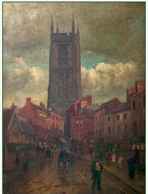
The tower of All Saints Church, Derby - now Derby Cathedral - in 1889, painted by Alfred John Keane (1864-1930)
